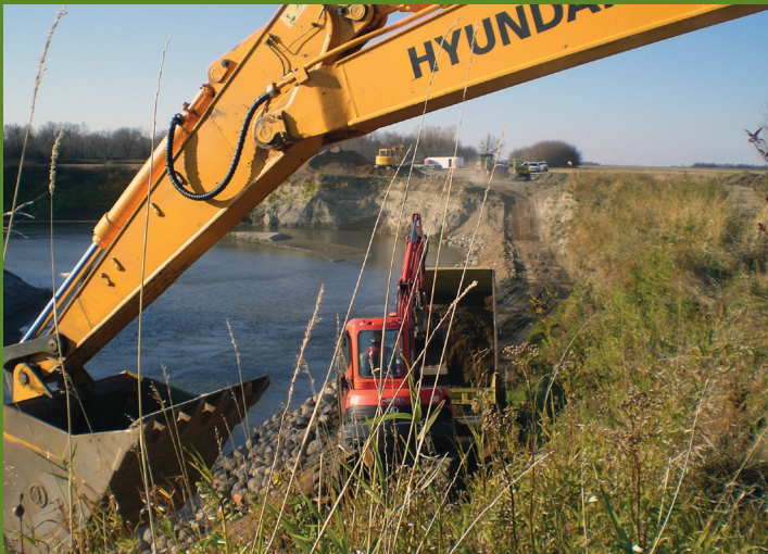
Northern Clearing crews start to lay the concrete armor.
